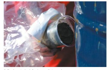
3. Push onto leak for immediate seal
