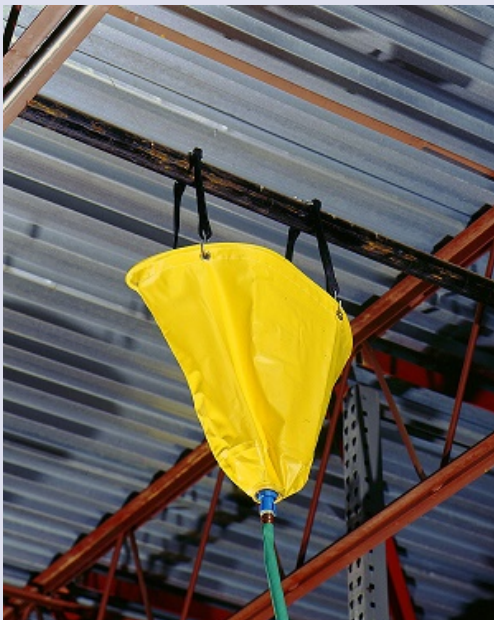
Pipe Drip Diverter
